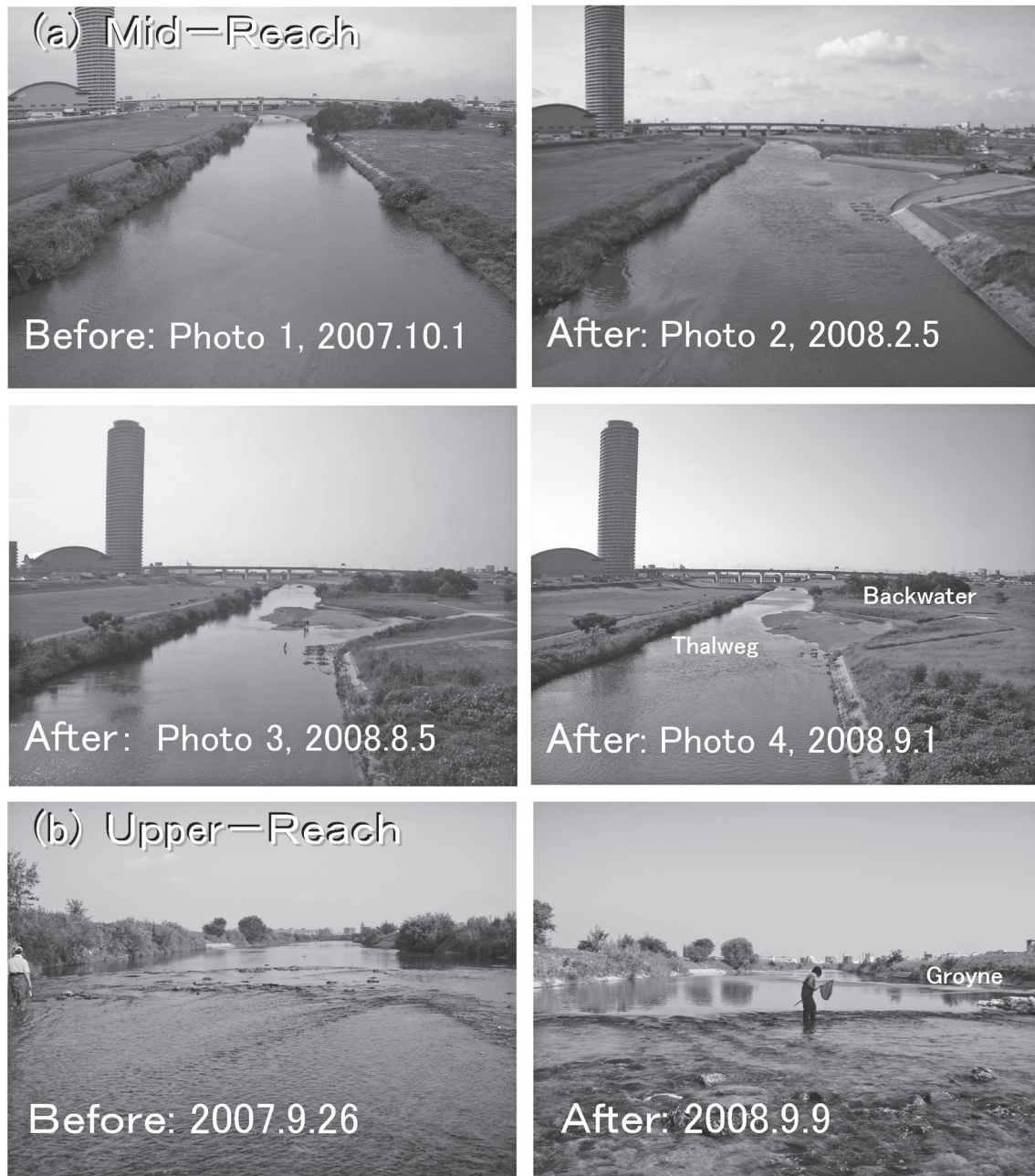
Fig. 4. Landscape changes observed from the fixed point at both the Mid- (a) and Upper (b) reaches before and after rehabilitation.
