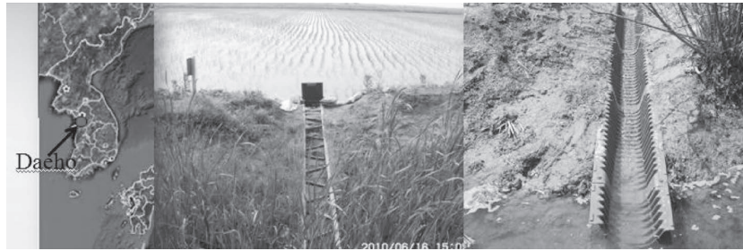
Fig. 10. Examples of fishway to connect between paddy field and irrigation canal.
